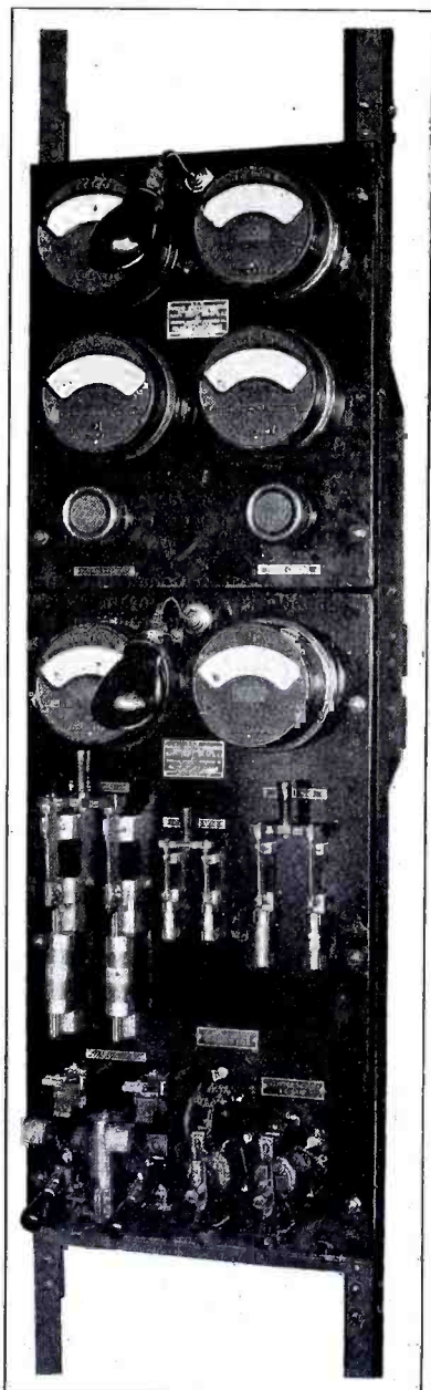
The Type of Switchboard Which Meets with Approval at all Radio Stations. Instant Control of Any of the Primary Circuits Can be Had.
